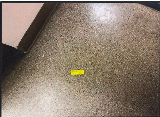
Photo #:5 Material #:5 Non-ACM Subject: View of Green Sheet Flooring w/ Red Pebble Design. Located in various rooms see table.
