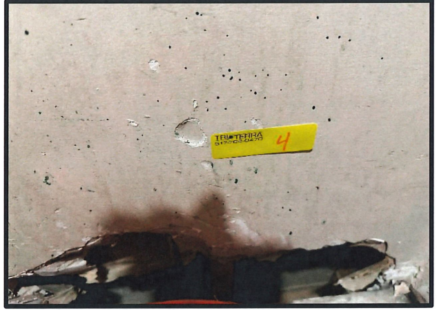
Photo #:4 Material #:4 Non-ACM Subject: View of Drywall w/ Joint Compound. Located on walls throughout.
