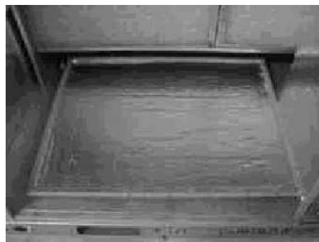
Figure 18: Return Downflow Plenum With Panel
