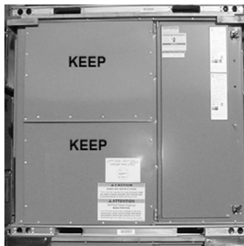
Figure 20: Save Side Panels For Economizer Hood Tops
