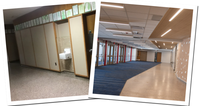
Before and after photos of the atrium at Everett. These are just a sample of the work, but the improvements are significant.
