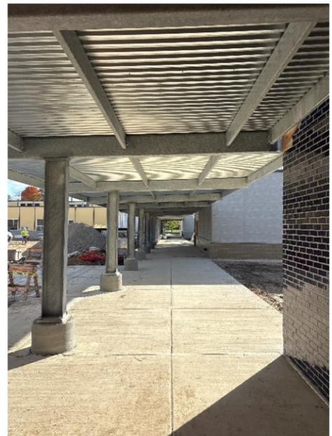
Covered Canopy Walkway Installation
