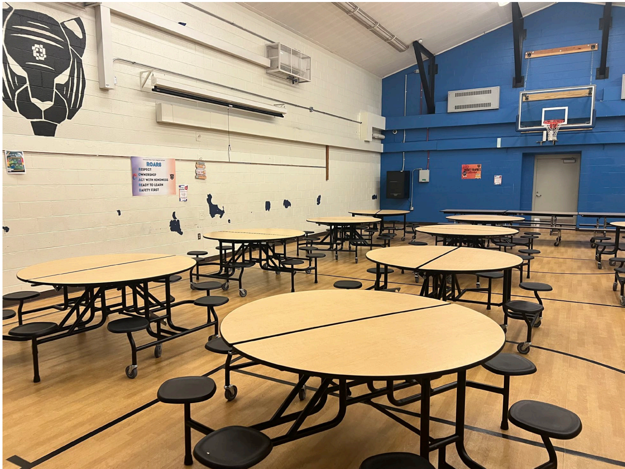
Figure 4: East wall Multi-Purpose Room
