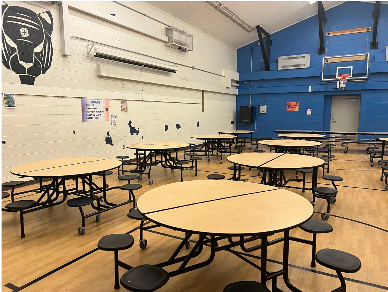
Figure 4: East wall Multi-Purpose Room
