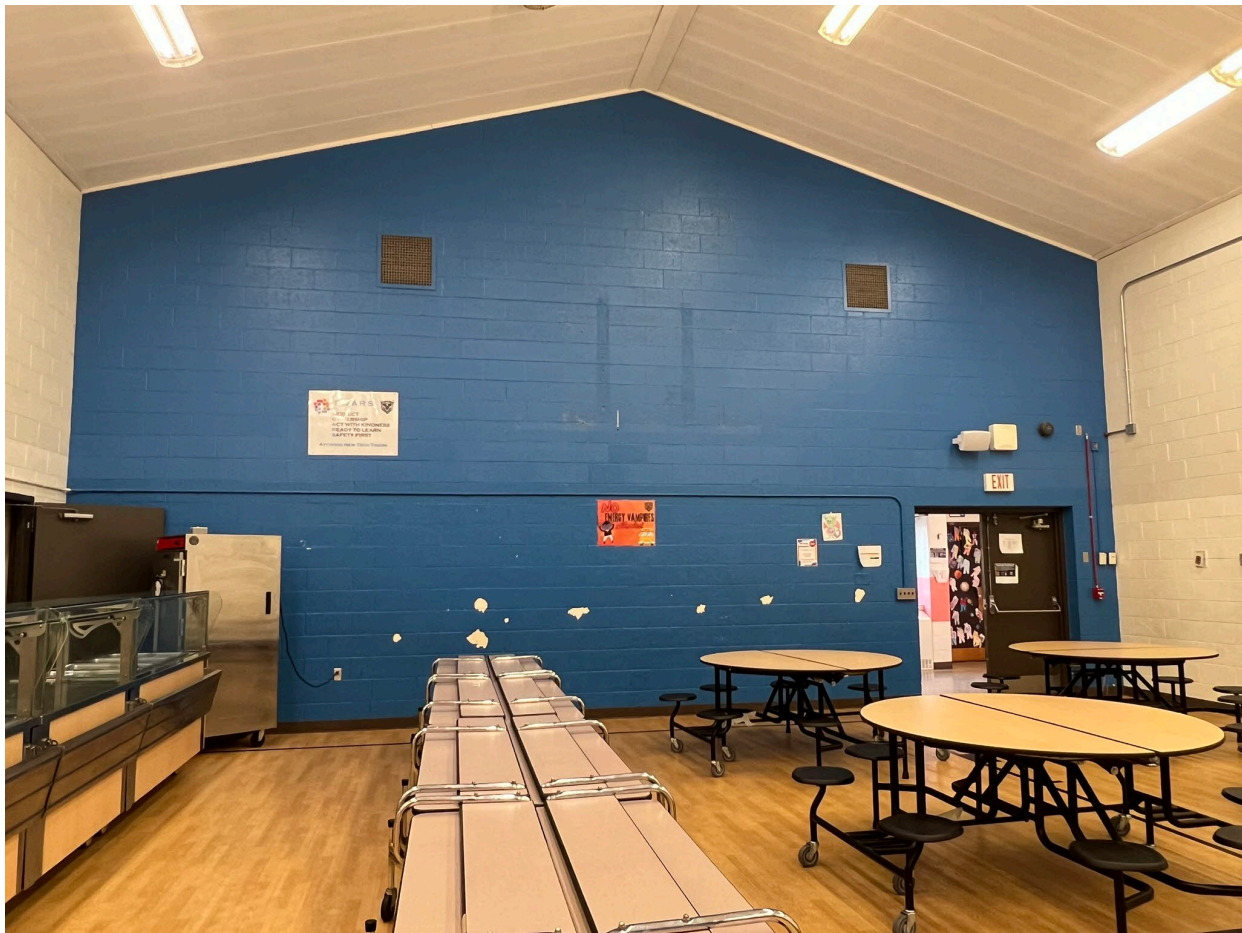
Figure 1: North wall Multi-Purpose Room
