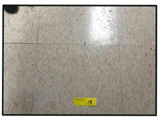
Photo #: 10 Material #: 13 **ACM** Subject: View of asbestos-containing 12"x12" tan VCT with brown specs.
